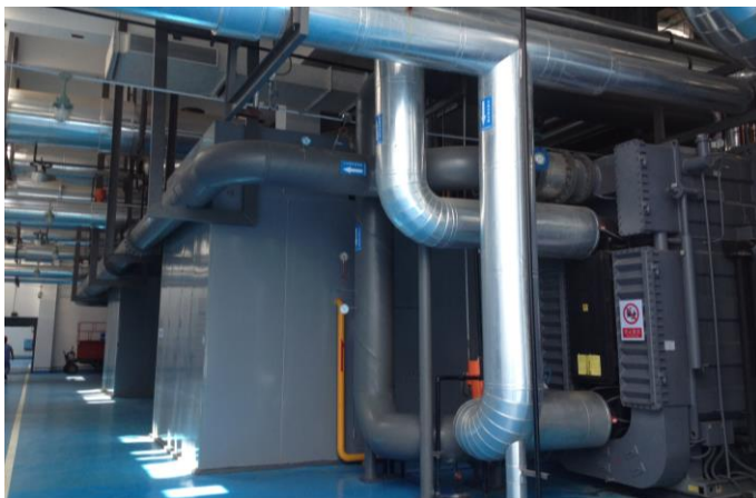
BROAD exhaust, hot water & direct-fired non-electric chiller
