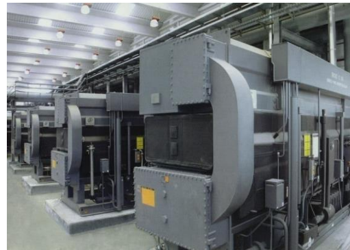
BROAD hot water type non electric chiller
