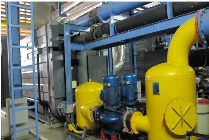
BROAD exhaust & hot water packaged chiller
