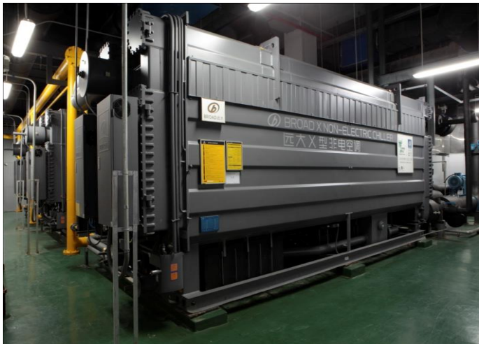
BROAD exhaust, hot water & direct-fired non-electric chiller
