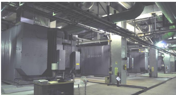
BROAD Exhaust, hot water & direct-fired chiller
