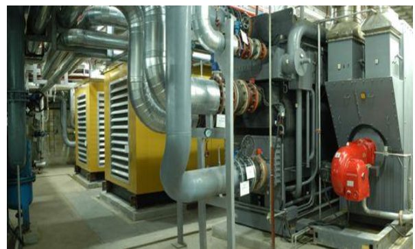
Gas engine & BROAD exhaust, hot water & direct-fired non-electric chiller
