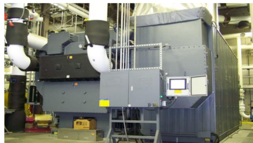
BROAD exhaust non-electric chiller
