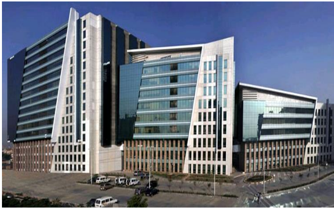
The world largest typical distributed energy system which was totally unaffected in India black-out in July, 2012
