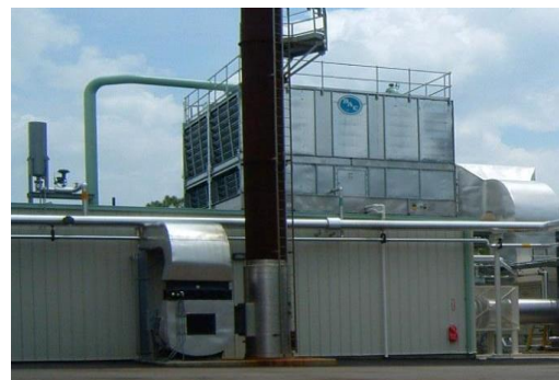
BROAD CCHP exhaust non-electric chiller
